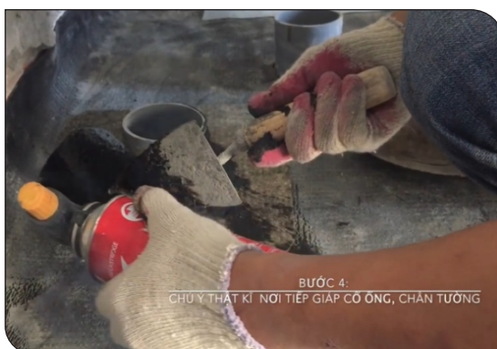
Treating the neck of the drain pipe
